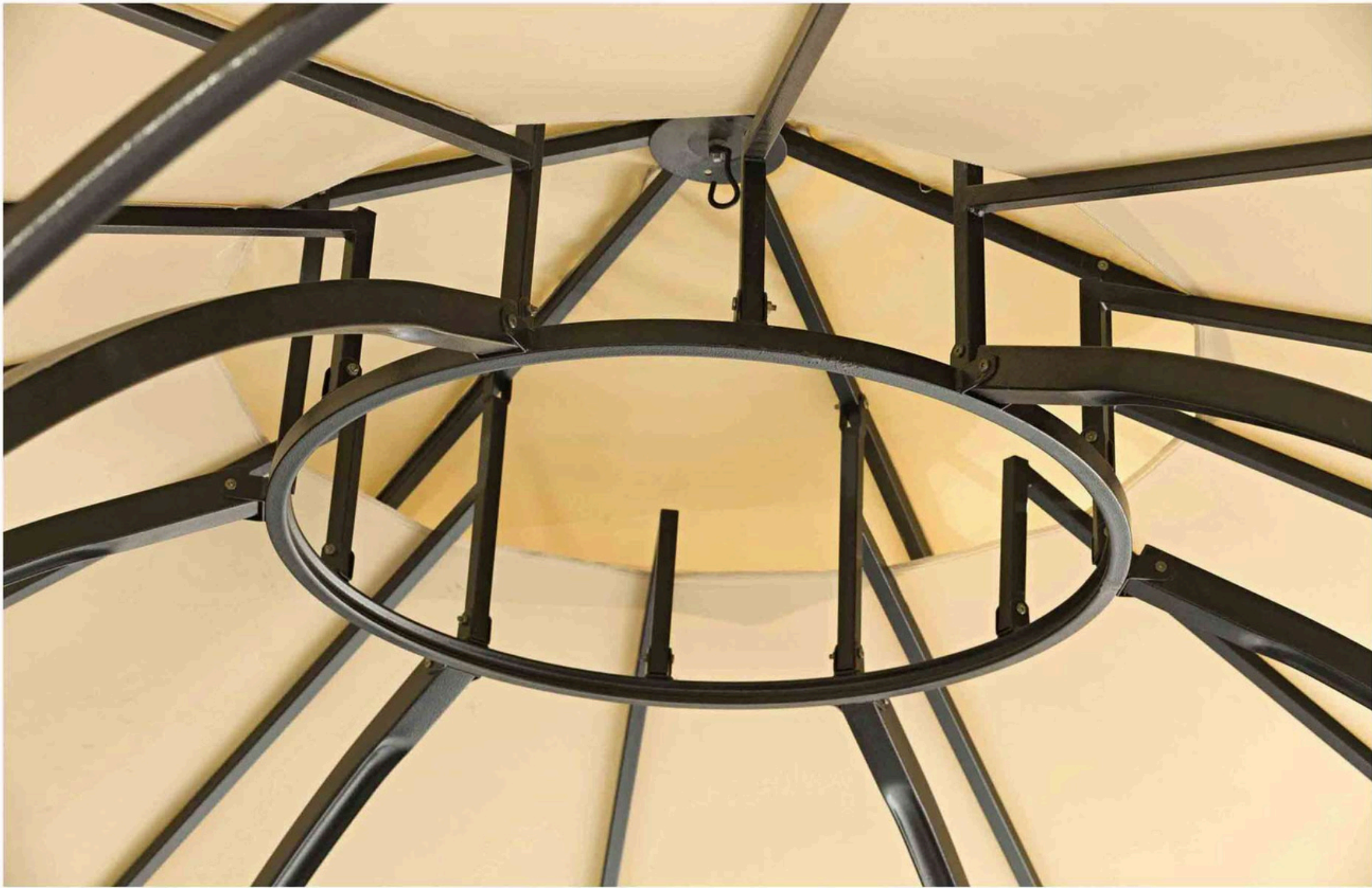
Reinforcement ring fixed in the shed
